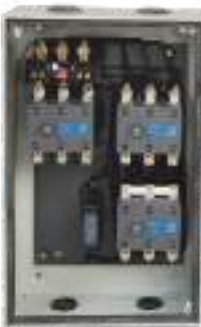
Interior View of ML FASD
