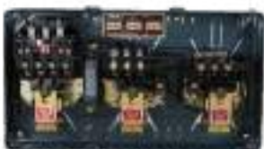
Interior View of MK1 FASD
