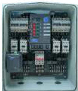
Interior View of xMU-GiA
